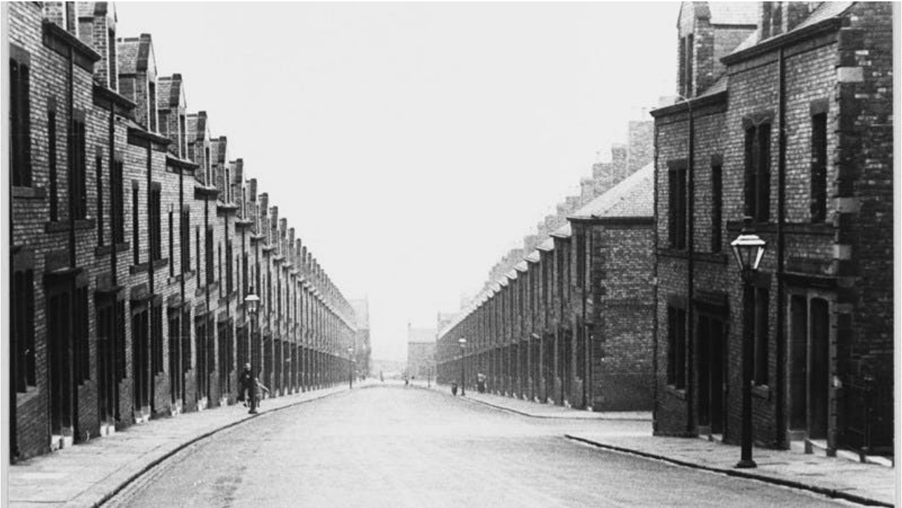
Early 19th century terraced houses
